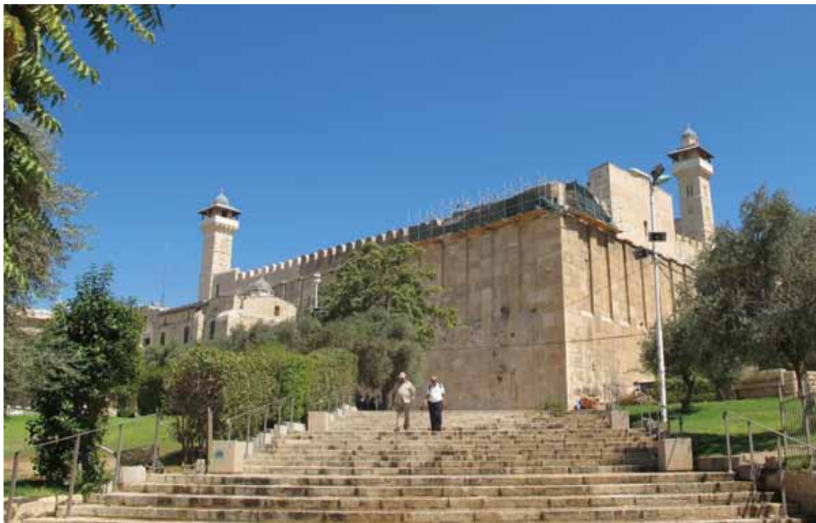
Image 8: These massive walls around the tombs of the patriarchs of Israel (see Gen. 23:9) in Hebron, a few miles south of Bethlehem, were originally constructed by Herod the Great (Matt. 2:1-23), who also rebuilt the temple of Jerusalem (John 2:20). (Image by user Ooman, courtesy of Wikimedia Commons.)
