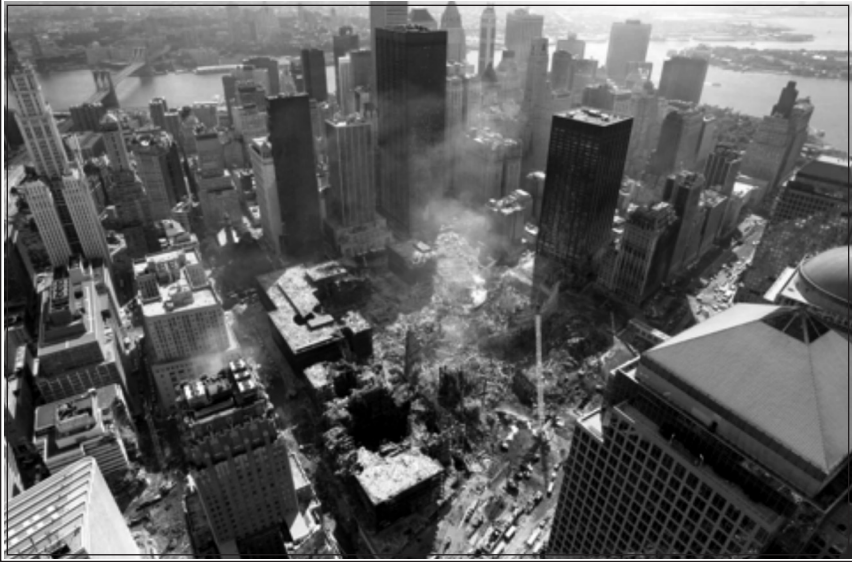
Ground Zero, seen from above. (Used courtesy of FDNY Photo Unit.)
